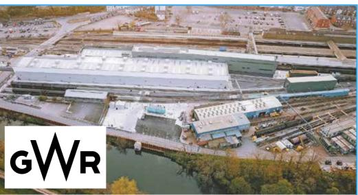
The new depot includes a three-road maintenance shed that comprises two five-car inspection/maintenance roads and a three-car heavy lift road.
